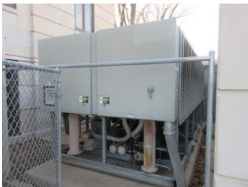
The existing chiller from 1999 at the Courthouse is reaching the end of its expected life and causes major noise issues for spaces near its location
