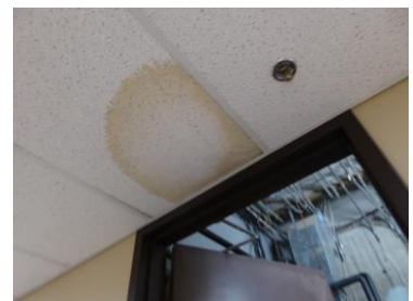
Numerous pipe leaks above the ceilings are problematic at the Law Enforcement Center
