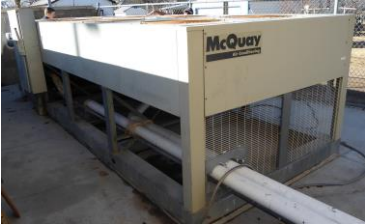
Air-cooled chiller that has had numerous major maintenance issues in recent years and is at the end of its life serving the Administration Building
