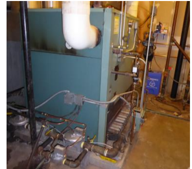
Low pressure steam boiler at the Library is a major source of concern for failure without any backup
