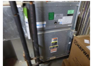
Reverse-cycle water source heat pumps in the Law enforcement Center cause major maintenance issues and are beginning to leak and fail
