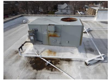
Rooftop units serving fourth floor at Courthouse are failing
