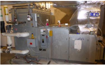
Ineffective and problematic multi-zone unit that does a poor job of providing comfort to spaces in the Administration Building
